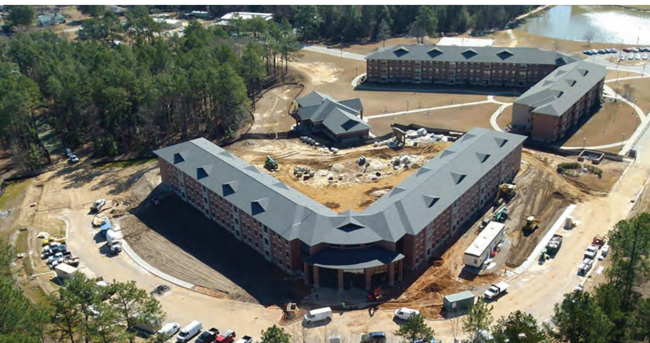
EGSC'S NEW RESIDENCE HALL, BOBCAT VILLAS - WEST, UNDER CONSTRUCTION
